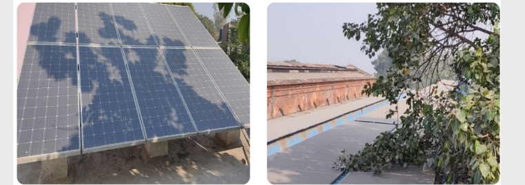
Low energy production due to shading
